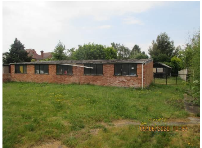
View of garages facing west
