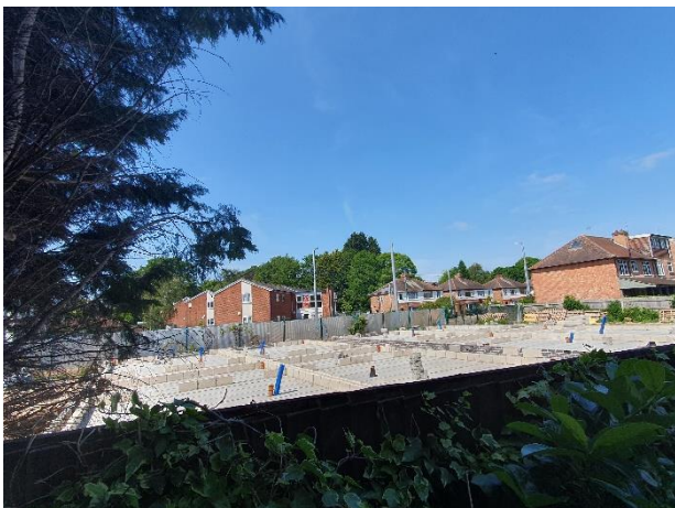
Wider site, permission being constructed under 21/01055/FUL – facing north west from rear footpath
