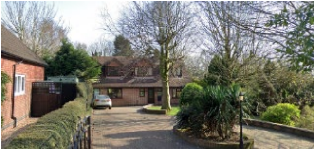
Front (north west) elevation and boundary with no. 105.
