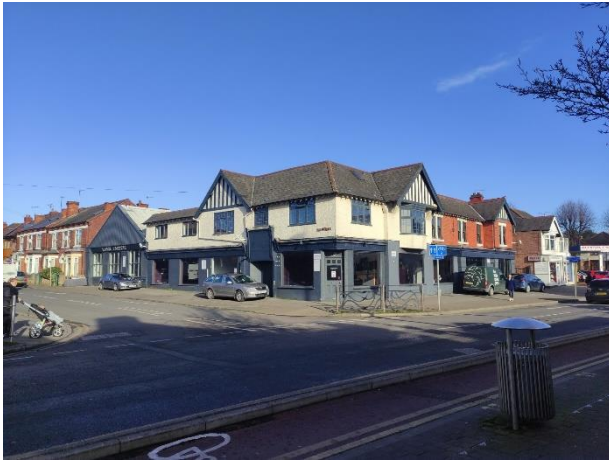
View from Marlborough Road/High Road
