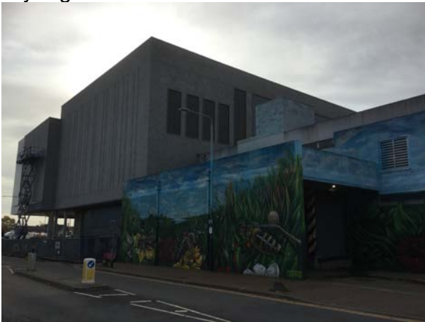
North west and north east elevation from Station Road
