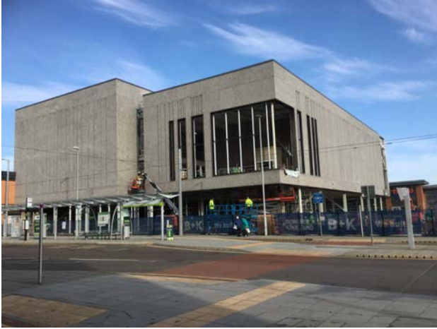
South west and south east elevations from Styring Street
